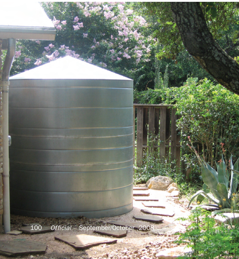
← A 2000 gallon galvanized metal cistern used for rainwater catchment for irrigation purposes. (Photo by IWS, watercache.com)
