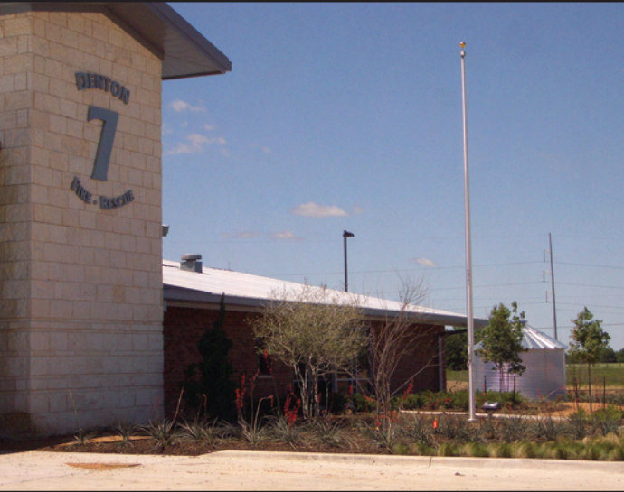
This rainwater collection system in Denton, Texas, helped the fire station achieve a LEED Gold rating. Rainwater is stored in four 5,600 gallon tanks and used to irrigate native plant landscaping around the station. All collection pipes were integrated into the concrete slab of the rainwater tank to give a very clean appearance.
