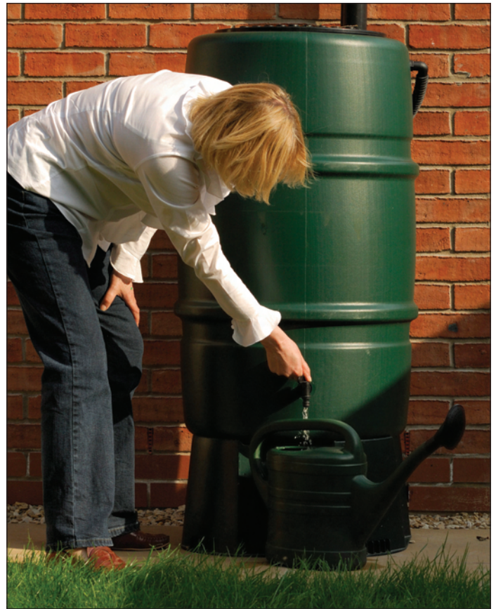
The simplest rainwater harvesting system is roof water draining into a rain barrel.
