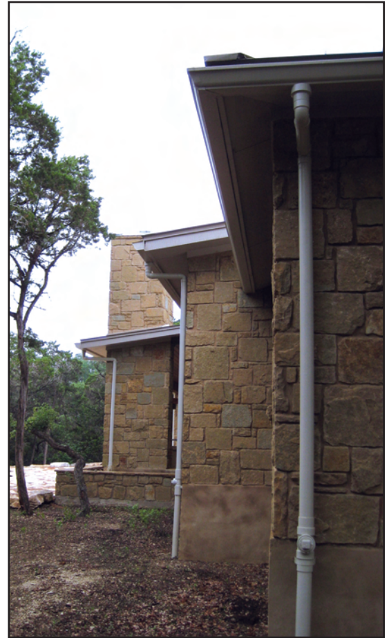
The downspouts connect to the underground collection piping and delivers the rainwater to the storage tank (by gravity, no pumps).
