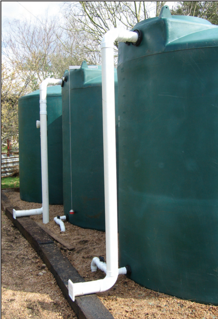
This hybrid system collects rainwater, but will switch over to the well water tank (furthest tank in picture) when the rainwater tanks run dry.
