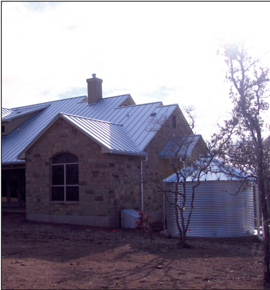
The downspouts connect to the underground collection piping and delivers the rainwater to the storage tank (by gravity, no pumps).
