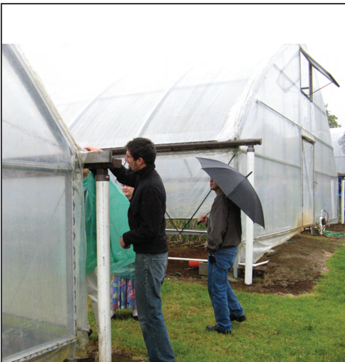
A rainwater collection system at a greenhouse.
