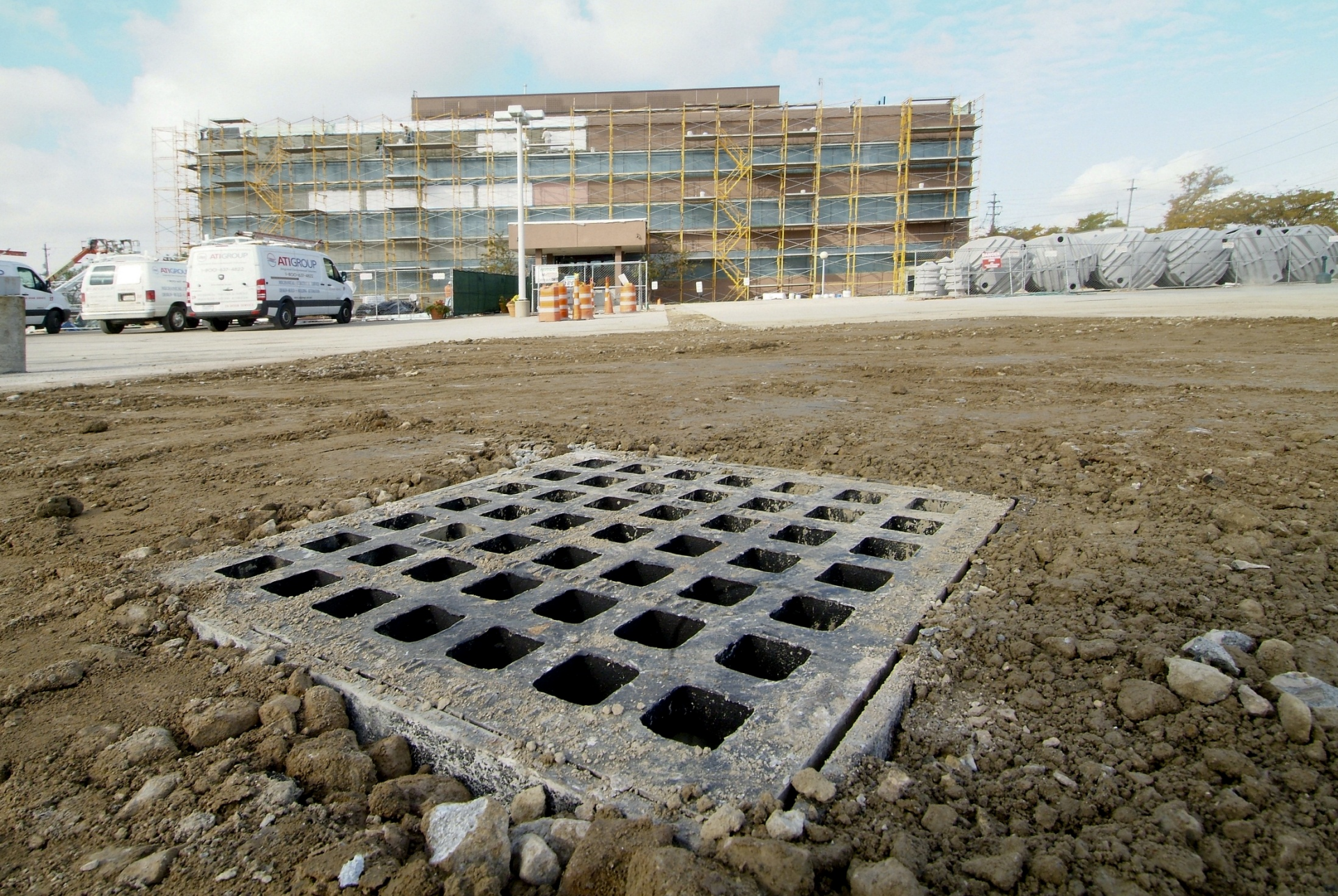
Completed installation of vault with 6 cisterns waiting for installation.
