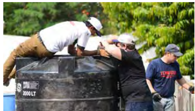
Members of Team India (Lalit Kasawate), Team Australia (Aaron Bridger), and Team USA (Adam Koenigs) work together on the school roof to install a new water tank that will supply the upgraded handwash area. Credit: Anill Patil
