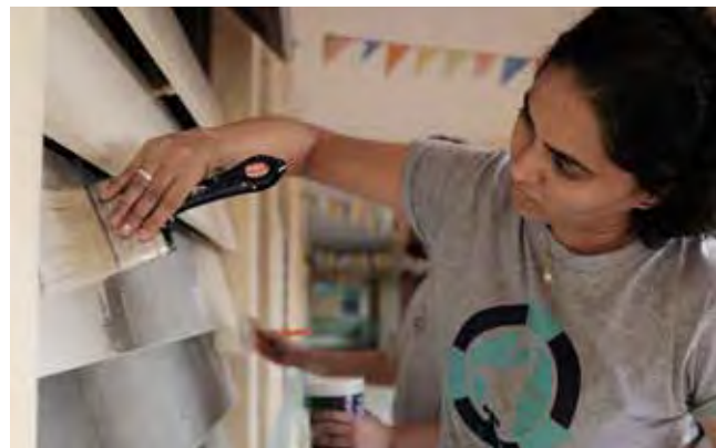
Swathi Saralaya of IAPMO India puts the finishing touches to new louvres added to help improve light, ventilation and privacy for the boys and girls toilets. Credit: Alan Gwee
