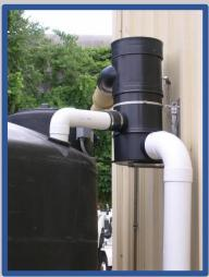
Sample self-cleaning rainwater harvesting pre-tank filter
